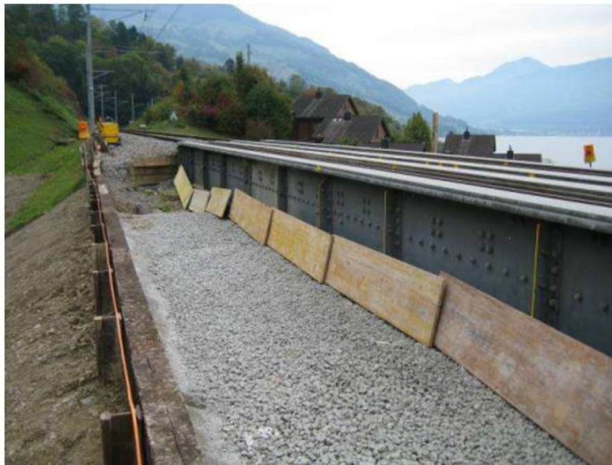
Temporary auxiliary bridges (real example)
